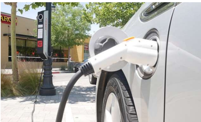
Street-Side Lamp / Power Pole
